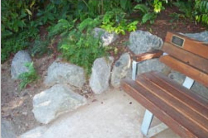
By installing the rocks first and then pouring concrete right up to the edge, E. J. Hook eliminated a common weed problem.
