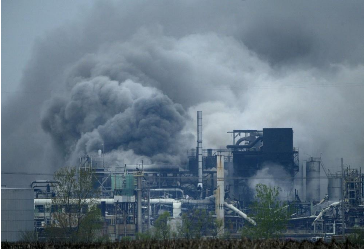
Vinyl Chloride Explosion, Formosa Plastics, Illiopolis, April 23, 2004. Chemical Safety Board photo.
