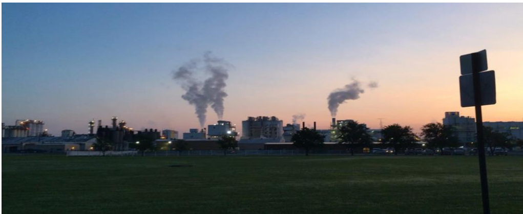
Westlake plant in Calvert City, 2019. Jim Vallette/Material Research
